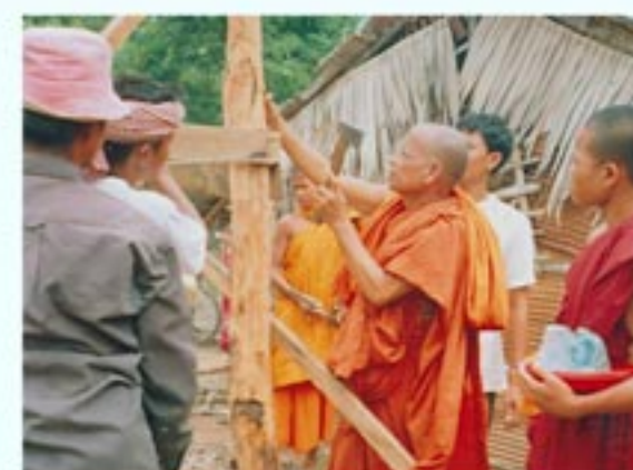
Monks are building a house for PLHIV family
